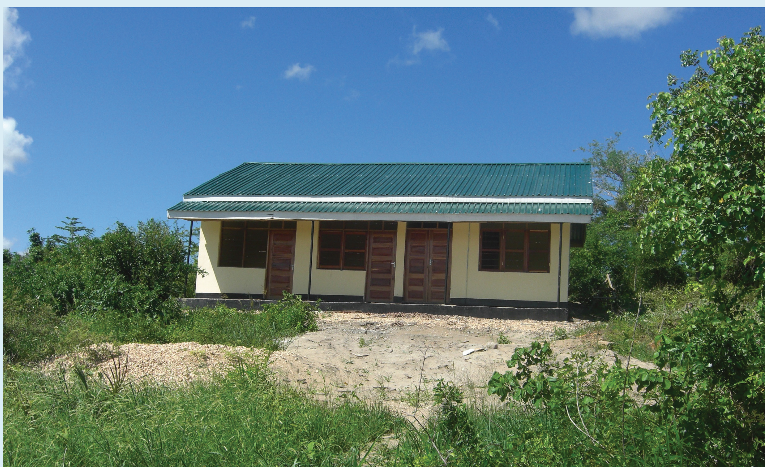
New village office in Pangani District, provided by the investor - case study A (photo: M. Locher 2011)
